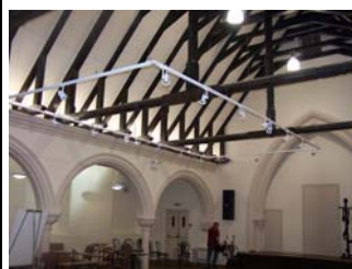
Refurbished Upstairs Hall
